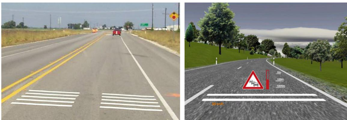
**Figure 3.22:** Picture of real rumble strips for speed reduction (left) and the implementation in the HUD (right). Several sets of rumble strips were installed upstream a construction site with small but statistically significant speed reductions (see [Mil+05]). Every time a virtual strip passes "under" the ego vehicle a rumble sound is produced by the subwoofer in the driver seat creating vibrations for haptic feedback (scene and HUD content digitally mixed).
