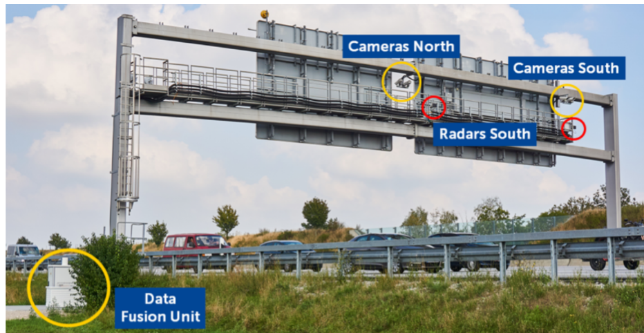
Figure 1.2: An image of a single Providentia measurement point on the A9 highway. Two optical cameras pointing in both road directions are visible (yellow circles on top). Two radars pointing to the south can also be seen (red circles). Also, a Data Fusion Unit (DFU) collecting and fusing the sensory data is displayed on the image in the bottom left corner.
