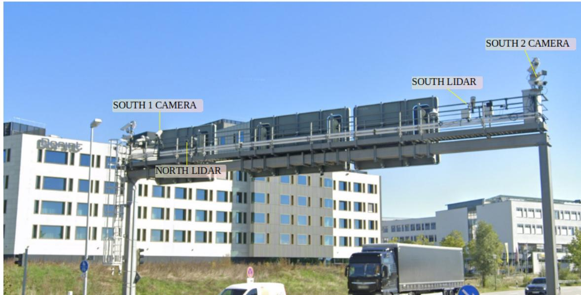
**Figure 3.2:** S110 gantry sensor setup. Image capture: Sep 2023 © 2024 Google
